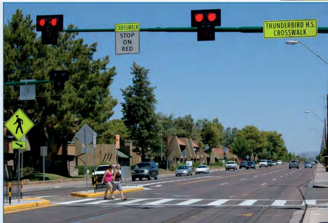
Figure 1. A PHB in Phoenix Arizona provides protection for pedestrians near a high school. Photo Credit: Mike Cynecki
