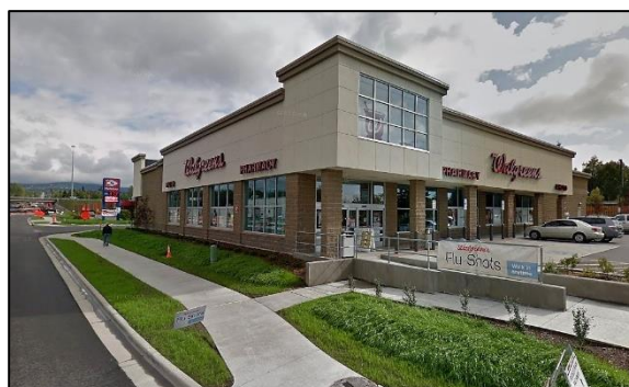
Commercial development with pedestrian-supportive street frontage.
