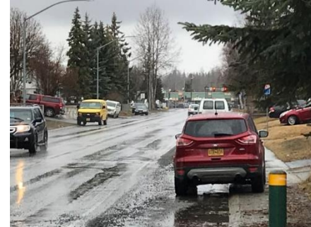
Parked car on a rolled-curb sidewalk.
