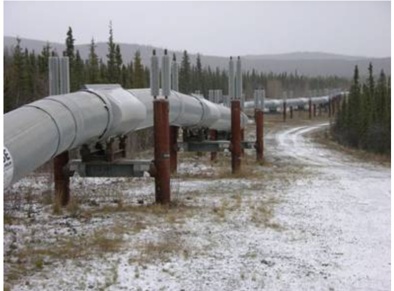
The Trans-Alaska Pipeline
