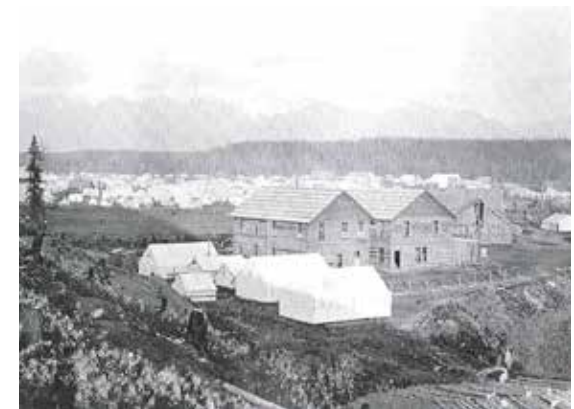
By 1915, Ship Creek was filled with over a thousand tents as the Alaska Engineering Commission began construction of the railroad.
