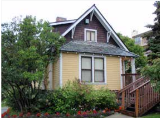
The Oscar Anderson House (1915) has consistently been identified through surveys and public outreach as one of the top “Landmarks to Save.”
