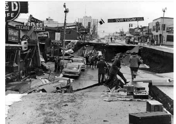
Fourth Avenue, damaged by the 1964 Good Friday Earthquake.
