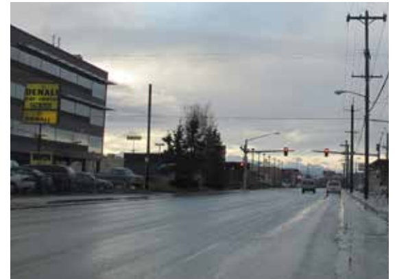
The Gambell-Ingra Corridor was once Fairview's "main street," but it now bisects the neighborhood.
