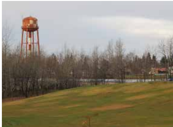
Green space buffers the hill from nearby industrial activity.
