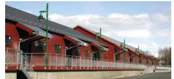
The Alaska Railroad Freight Shed is LEED-certified and listed in the National Register of Historic Places.
