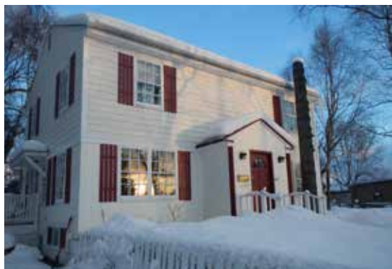
Prioritize nomination of National Register-eligible properties outside of Downtown, such as these CAA/FAA Duplexes in the South Addition.
