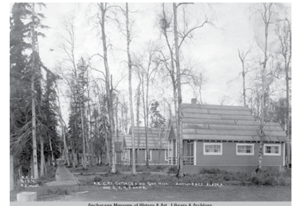
Alaska Engineering Commission (AEC) Cottages on Government Hill, 1916.
