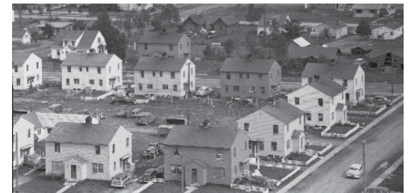
Detailed view of CAA duplexes at 13th Avenue and I Street from roof of 1200 L Street, 1951.
