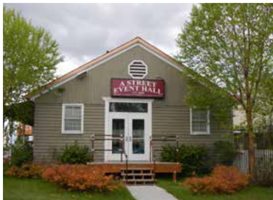
Historic buildings can be used as community meeting places, such as the A Street Event Hall in Downtown.
