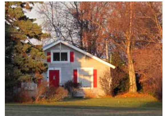
Strutz House, P Street.
