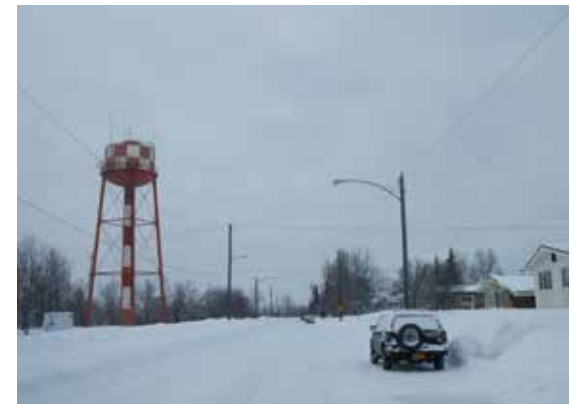
The Government Hill Water Tower is a neighborhood icon in all seasons.
