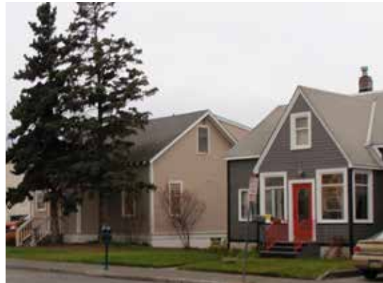
AEC Cottages on 3rd Avenue (listed in the National Register).
