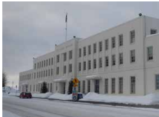
Alaska Railroad Passenger Depot.
